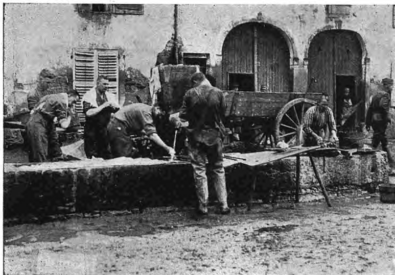
MODERN IMPROVEMENTS AT NEUFMAISONS
