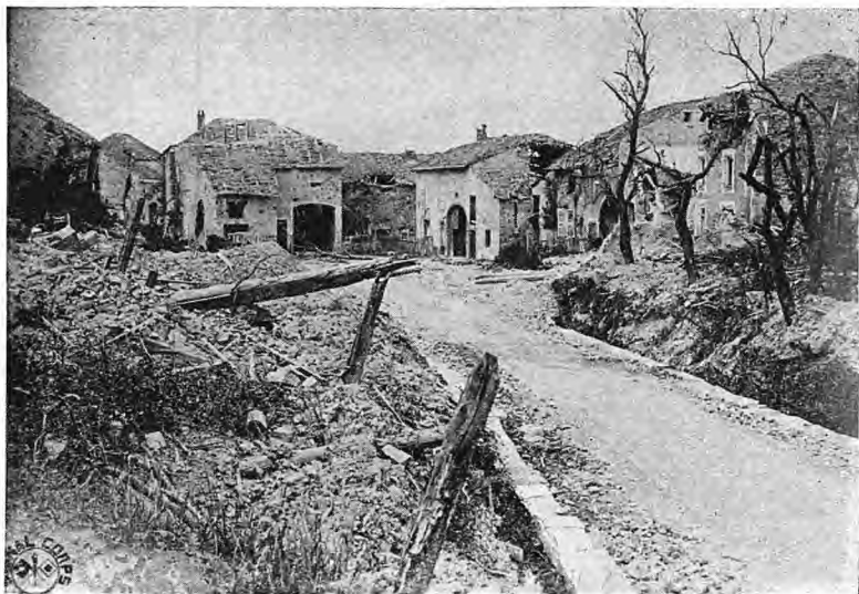
LOWER PART OF BADONVILLER WRECKED BY SHELL FIRE
