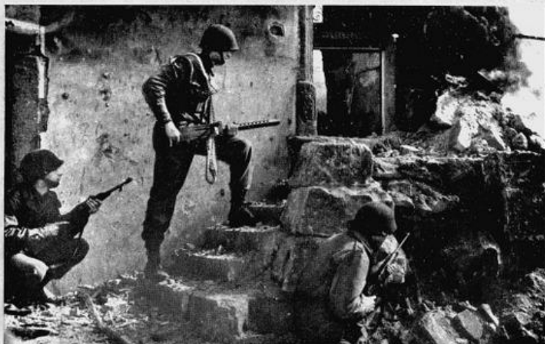
HOUSE TO HOUSE CLEAN-UP
