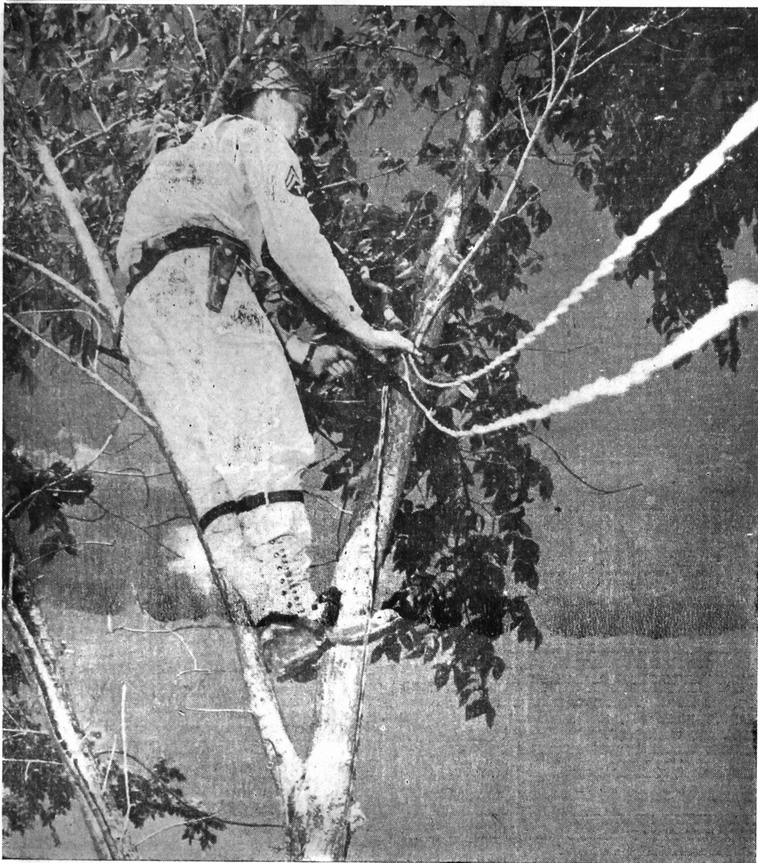
If this were a scene taken in a combat area, and the enemy was anywhere near, two men would be on the ground beneath this tree to watch for snipers while Pfc. Thomas G. Pleasant worked. He is shown here making a field wire tie, tying in two circuits. When wire is laid on the ground, it is snubbed around small stumps or trees at regular intervals to avoid having too much slack in the line.
