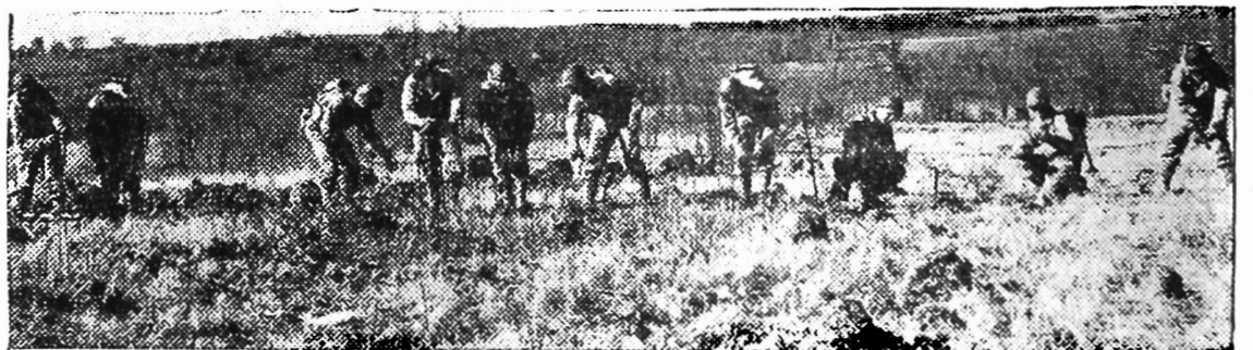
Squad from Co. B, 142nd Engineers, shown constructing a double apron barbed wire fence preparatory to blowing it up in a demolition problem.
