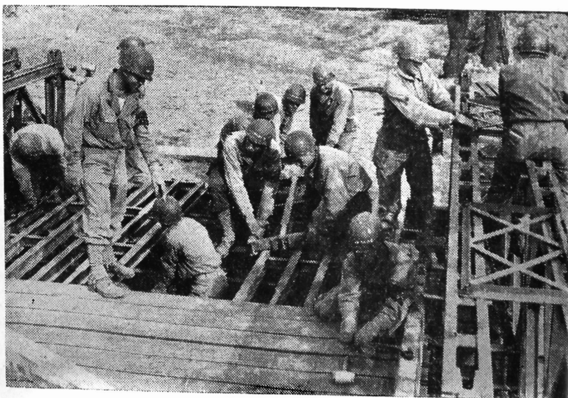
Members of Co. A, 142nd Eng. Bn., (top) push a completed section of a Bailey bridge out over the stream bed during a session in bridge building. This is just one of the many types of work done by the Engineer Battalion. (Right) the bridge nears completion as these men lay the last few pieces of foundation and cross pieces of the roadway on the bridge.
