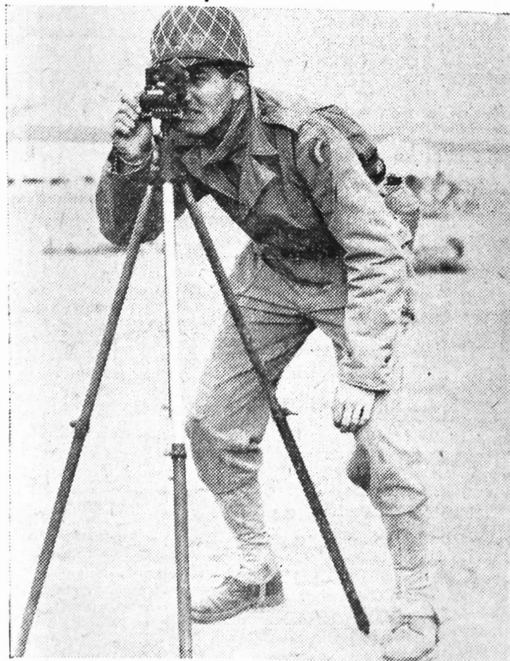
When the heavy weapons company goes into action one of the important men in getting the weapons on their targets is the instrumental corporal who uses the aiming circle and range finder. Above, Pvt. Edward Still, Co. M, 232nd Inf., takes a reading with the aiming circle.
