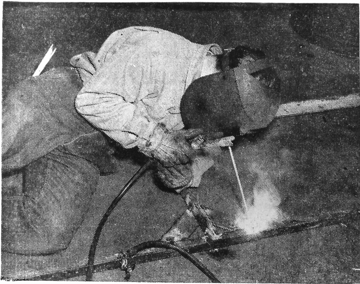
Framework for a stand on which a cabinet in the parts truck will rest is being welded by T-4 Weldon Carpenter in the welding department of the 742nd Ordnance Company shops. (U. S. Signal Corps Photo.)
