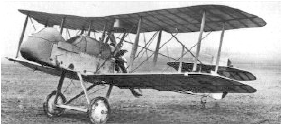
WWI-152 AIRCO DH2, which shows the progress toward an enclosed fuselage in the very early years of WW I.
